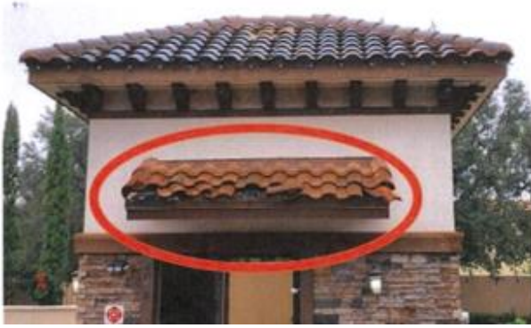
Guard Gate roof tiles - Before
