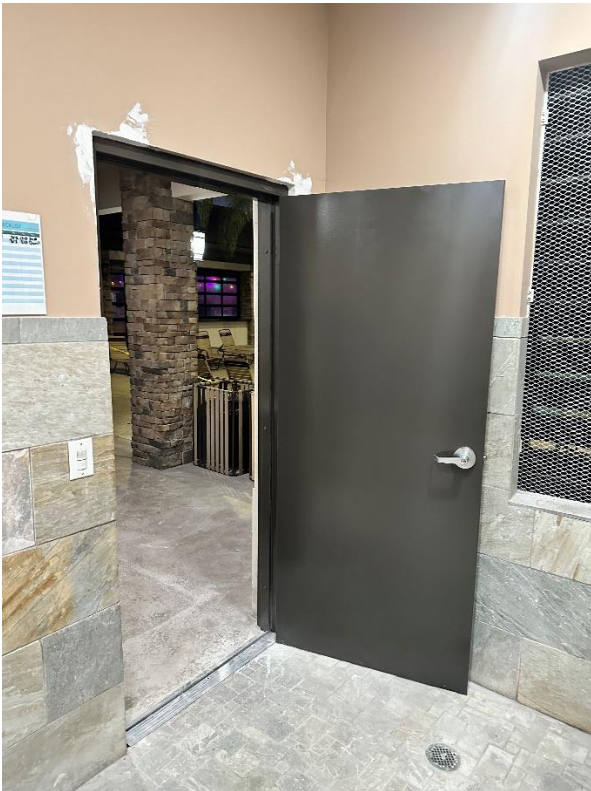
Outdoor Pool Restroom Doors - Complete
